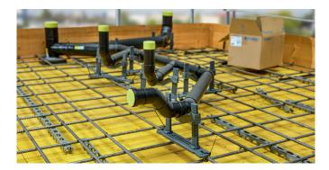
Planning a drainage system with the horizontal connection pipes in concrete floor, planners can now integrate the new Geberit cast-in-concrete brackets directly within the schematic planning module.
