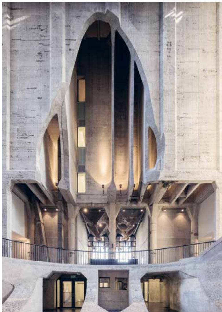
↑ Carved out of individual tube chambers, the atrium – which measures 4,600 m 3 – is modelled on a grain kernel.
