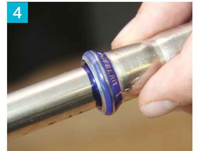
Insert pipe into fitting
