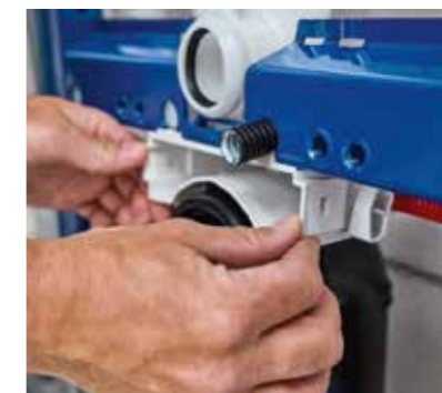
↑ A protection box ensures that the box remains clean during construction work.
