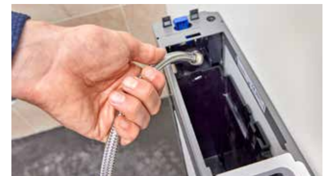
↑ The reinforced braided hose for the water supply connection can be built in without having to remove the flush water tank – that's one less step.
