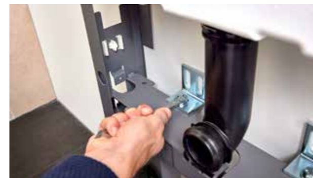
↑ Tried-and-tested mounting brackets are used to fasten the frame to the building structure.
