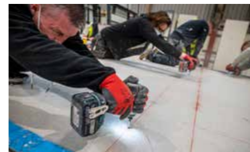
↑ First stage of construction.
